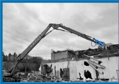
Okada TSRC Crusher-Shears are designed for the demolition of concrete-encased steel structures. Constructed entirely from cast steel, all TSRC models offer outstanding strength while minimizing weight. The cast steel body enhances durability by resisting stress-induced cracking and ensures a lighter attachment for improved carrier performance.
