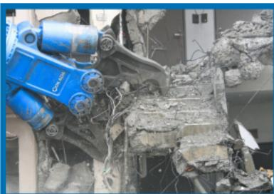
Okada's wide product range of TSW crushers give you a concrete solution for your carrier. All Okada TSW crushers are built from cast steel, providing exceptional strength without added weight. The cast steel body helps prevent cracking under stress while keeping the attachment lighter for better carrier efficiency.
