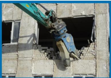
ORC series has an added rotator, built with a durable bearing. These rotating pulverizers allow you to process concrete wall, brick, concrete lumps into small pieces at great speed.
